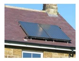
Happily the roof faces due south. To optimise the solar thermal energy collected and stored, the eco-house has a 300 litre dedicated solar tank. (A rule of thumb for optimal collection is 70 litres of tank per square meter of panel). Rather than being used directly for the hot water, the solar tank is used as a pre-heater for the thermal store.
