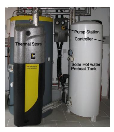
Whenever hot water is demanded in the house, the thermal store is topped back up by the solar water. If it has been a long sunny day, the large tank can reach over 60 °C and this hot water refills the thermal store for free. Even on a less sunny day, the solar tank will get to at least 40 °C, saving the heat pump from heating the water from cold. The beauty of this is that all heat losses from the solar tank are made up purely by the sun.
