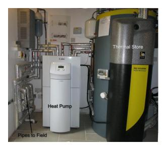
Cooler liquid at the bottom of the thermal store is circulated through the under-floor heating pipes to keep the house toasty-warm.
