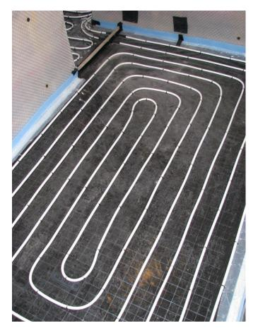
The eco-house opted for under-floor heating (as shown above). This method of heating warms the body from the toes up, so we feel warmer, and the thermostat can be lowered 1-2 degrees for the same comfort level.
