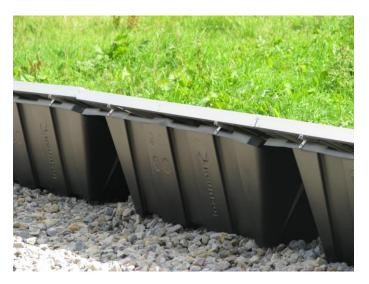
These, and the gravel base, were 'low carbon' compared with the alternative of aluminium roof frames, or ground frames on a concrete base (aluminium and concrete release CO<sub>2</sub> in manufacture).
