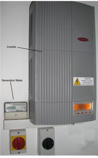
Installing PV is not a D-I-Y job for two big reasons. Firstly, this is potentially dangerous high voltage work and must be installed by an accredited Microgeneration Certification Scheme (MCS) member. Secondly, if you don't use an MCS installer, you won't get the feed-in tariff!
