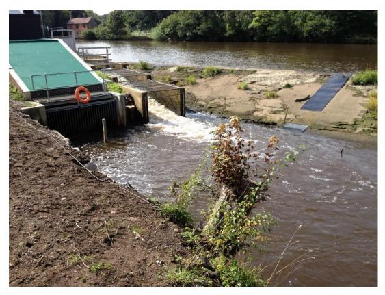
Figure 5. View of the new Larinier fish pass entrance, outfall of the new turbine and hydrophones array in 2013 with the hydropower scheme inactive.
