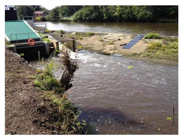
Figure 4. View of the Larinier fish pass entrance, hydropower outfall and hydrophones array showing the approximate positions of all 8 hydrophones in 2013.
