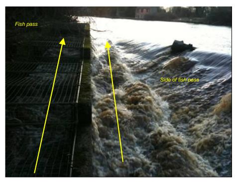
Figure 9. Old fish pass and side of fish pass ascent routes in high flows (35.9m<sup>3</sup>s<sup>-1</sup>) looking upstream. Arrows represent direction of fish passage (photo taken 3/1/2012 12:00).
