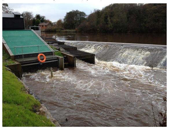
Figure 46. View of the outfall of the new turbine and hydrophones array in 2013 with the hydropower scheme active under higher flows.
