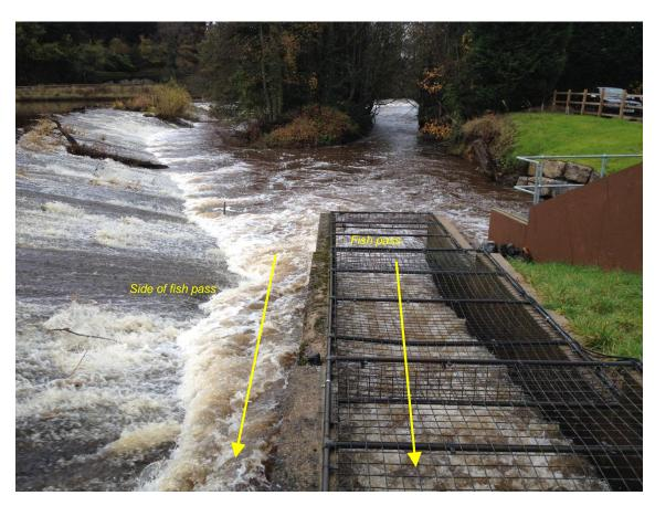
Figure 8. Larinier fish pass and side-of-fish-pass ascent routes, looking downstream. Arrows represent direction of fish passage (photo taken 22-11-2013 13:10).
