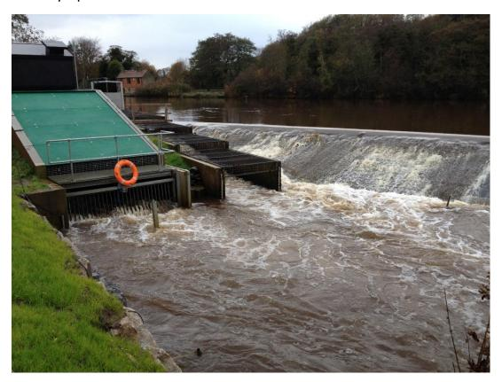
Figure 6. View of the outfall of the new turbine and hydrophones array in 2013 with the hydropower scheme active under higher flows. This figure highlights the visually more turbulent plumes of the fish pass and the left-hand side of the turbine outfall.
